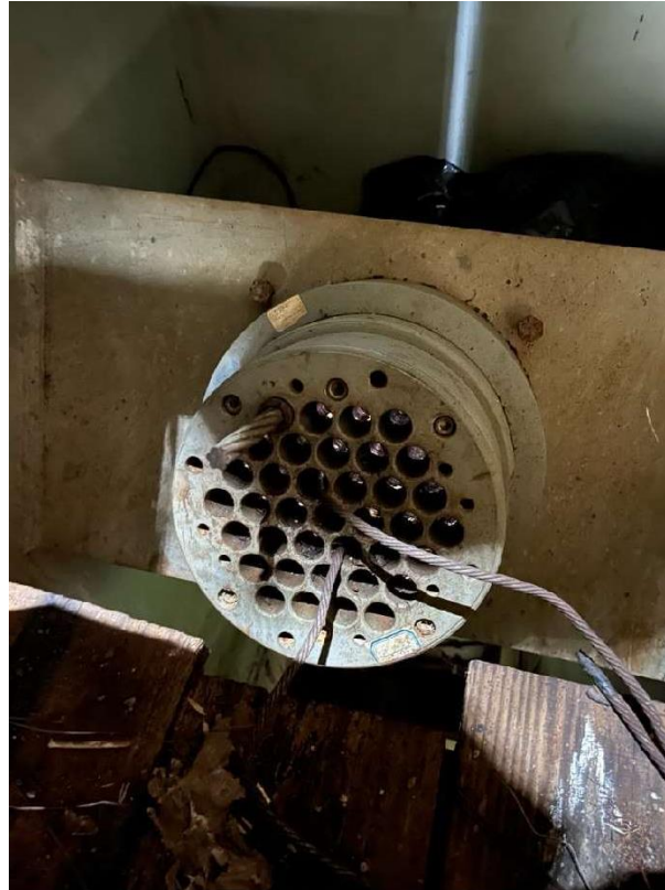
STRAND LOCKED ON PYLON END
