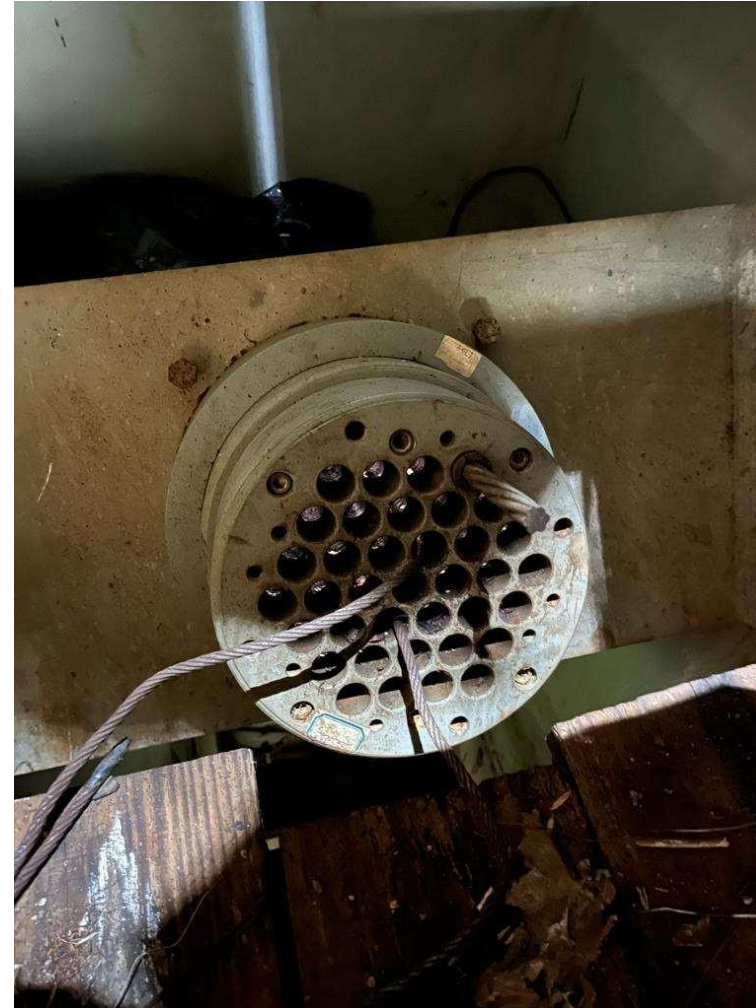
STRAND FIXED ON PYLON END
